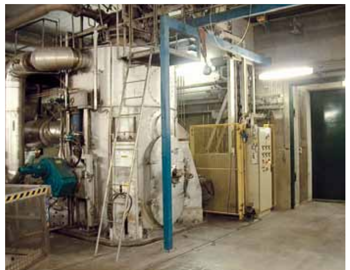
Armoured furnace for thermal disposal
